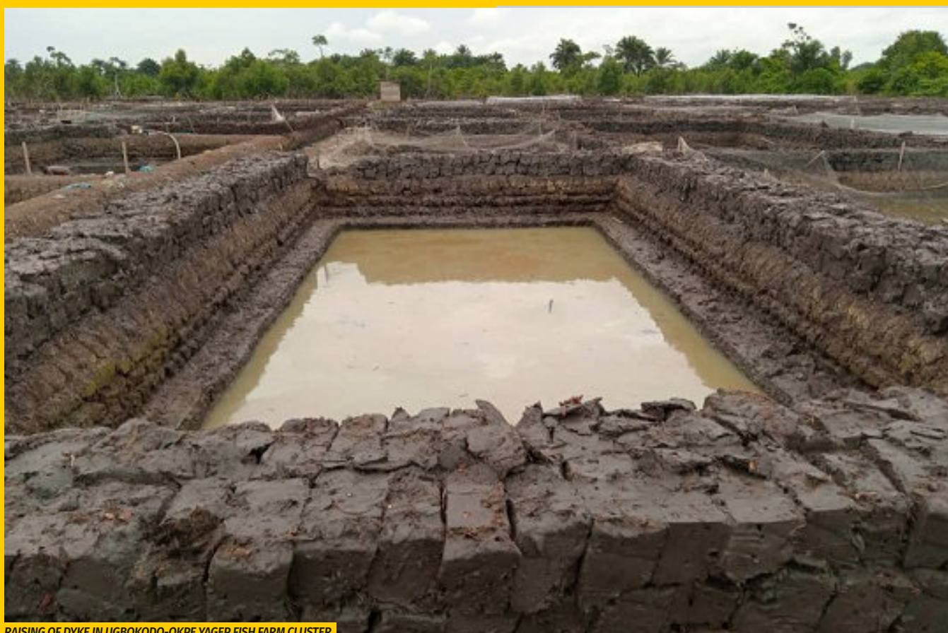
RAISING OF DYKE IN UGBOKODO-OKPE YAGEP FISH FARM CLUSTER
